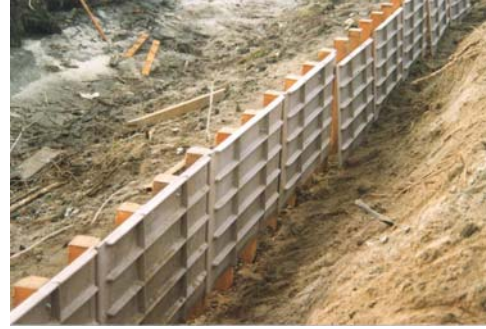
Fig 19 River Bank Protection
