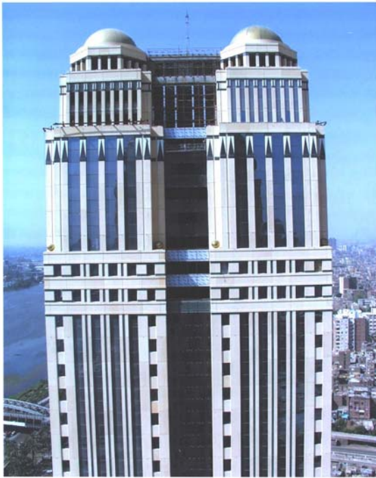
Fig 8 Nile City project, Egypt. 2 x twin Towers
