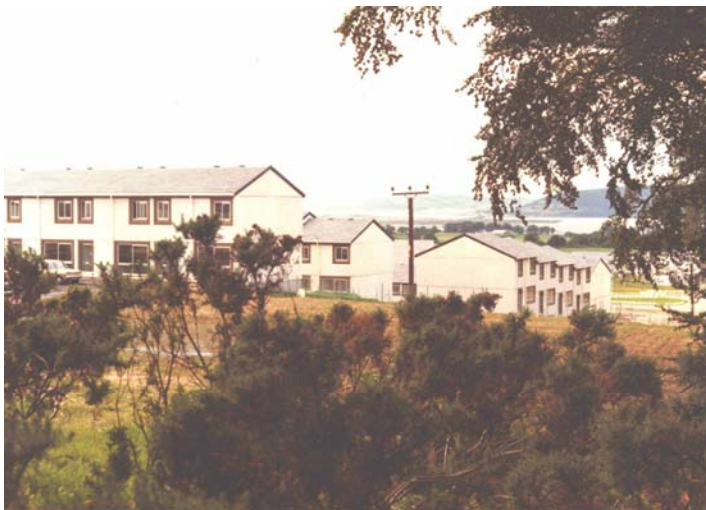
Fig 6 Timber Frame Houses with Single Skin GFRC Panels. Built 1976 UK
