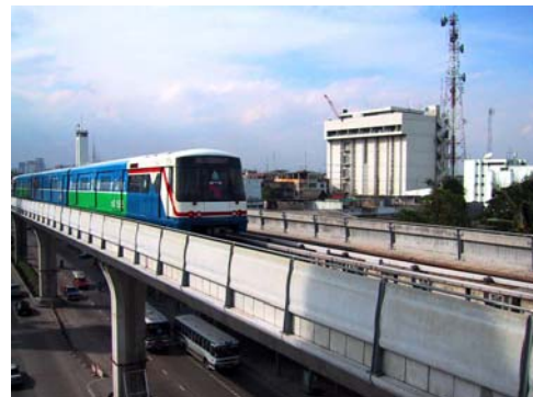
Fig 21 Bridge Parapets, Thailand
