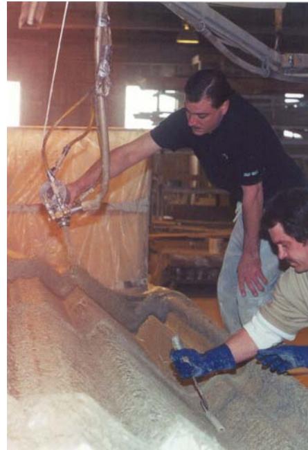
Fig 2 Simultaneous Spraying of GFRC
