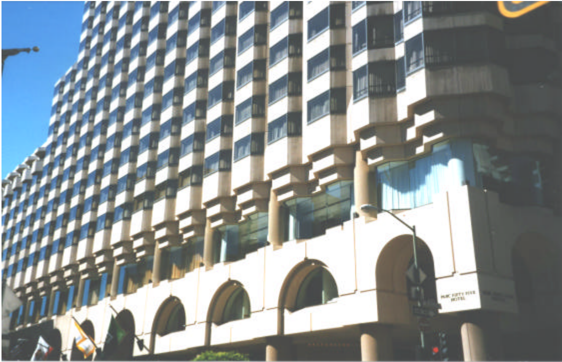
Figure 4: Parc Fifty Five, San Francisco. A variety of sculptured panels were created in GRC – from fluted, circular and oval column covers to delicately combed, three-dimensional spandrel panels and large arches with deep rustic joints: 3624 GRC panels cover 17,000 m 2 in total.
