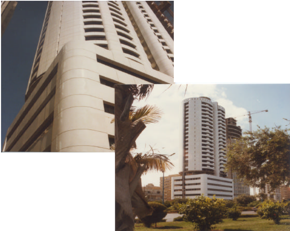
Figure 6: Corniche Towers, Abu Dhabi: nearly 10,000 m 2 of GRC has given 20 years of trouble-free performance in the Middle East's hot, salty and sandy environment.
