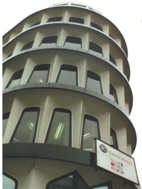
Figure 3: The light weight of GRC panels allowed this building in the City of London to incline outwards by 5 degrees thus increasing usable floor space. Nearly 30 years on, it is still a landmark building in excellent condition.
