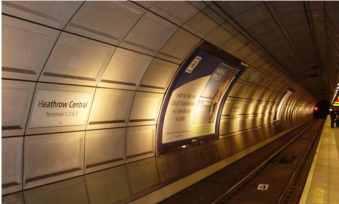
Fig 8 “Heathrow Express station lining panels”
